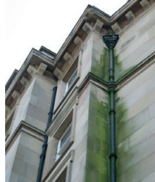
Leaking downpipe is causing damp and algae growth, which will erode the stonework
