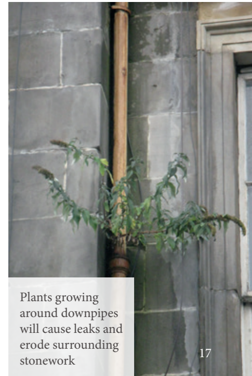
Leaking downpipe is causing damp and algae growth, which will erode the stonework
