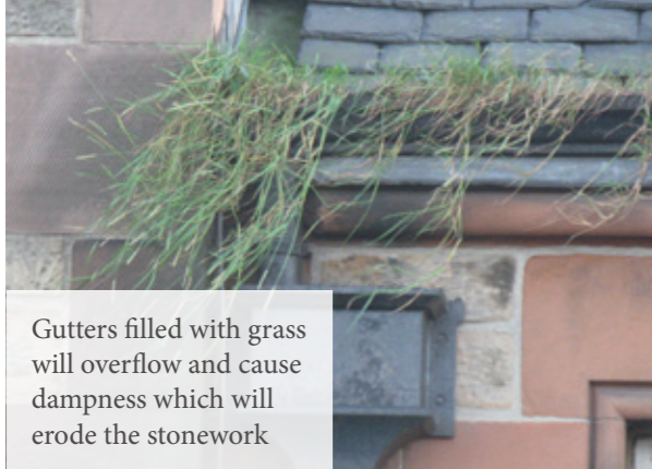
Downpipe is in poor repair causing leaking, damp and algae growth
