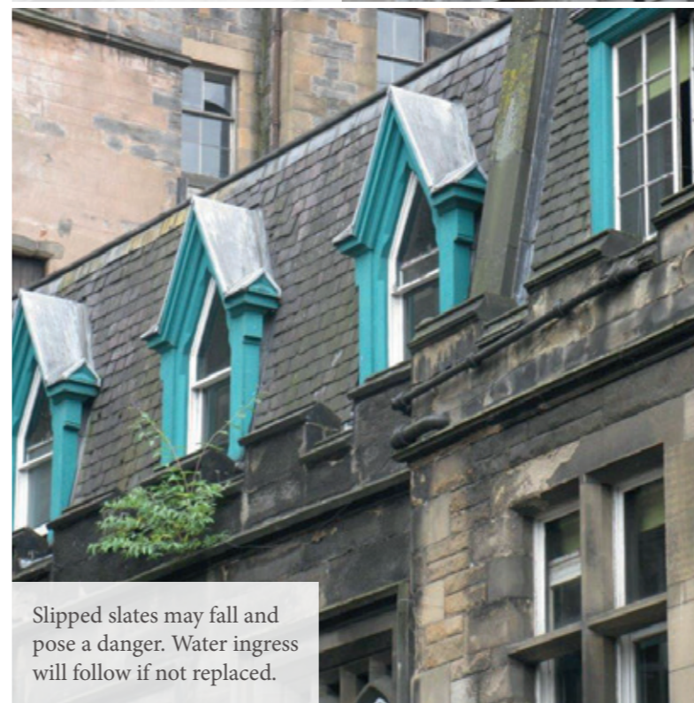
Vegetation has started growing on this stone ledge. If not cleared the ledge will decay.
